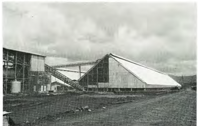
The 80 000 t capacity limestone storage building.
